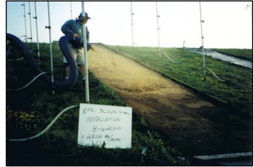
Figure 6. Blown Straw Installed for Testing
